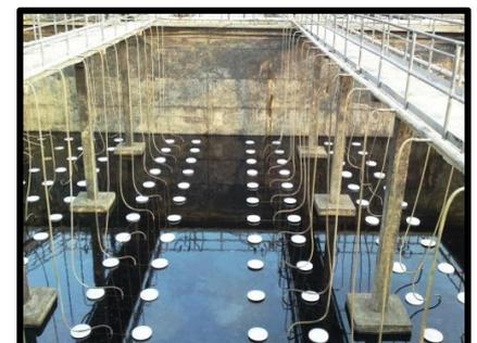
**Figure 4: Improved aeration units being installed throughout the BPC-ACT aerobic reactor**
