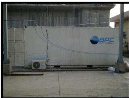
Figure 5: BPC-ACT skid mounted control unit installed on site at IOR
